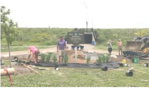
Work in progress for the President's Project!!
